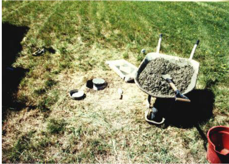
Concrete Mixed to Finish Hole Note, Area Kept Clean
