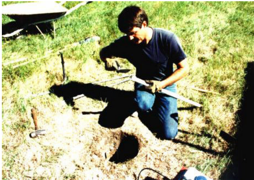
Preparing 1" PVC Greased Filled ("Finned") Sleeve
