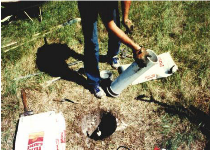
Gluing Logo Cap to 5" or 6" PVC Pipe
