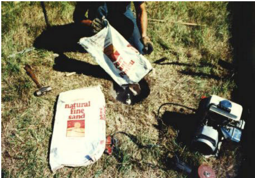
Backfilling Bottom 2 Feet of Hole with Washed Sand
