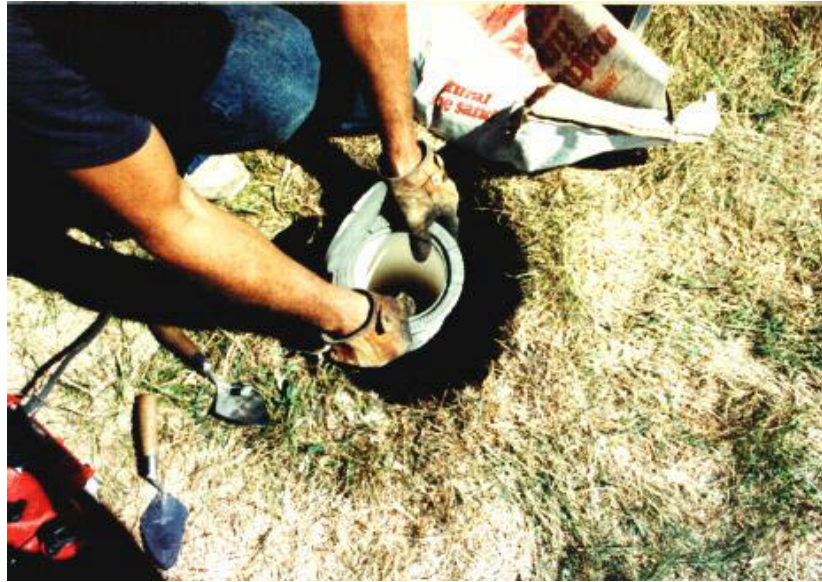
Placing Bottom of 24" Long, 5" or 6" PVC Pipe Into the Sand
