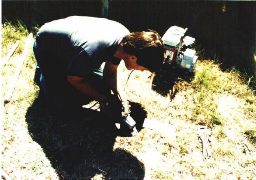
Rounding and Smoothing the Top of SS Rod with Grinder
