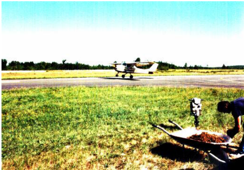
Finishing 12" X 48" Hole (Note, Safe distance from runway)
