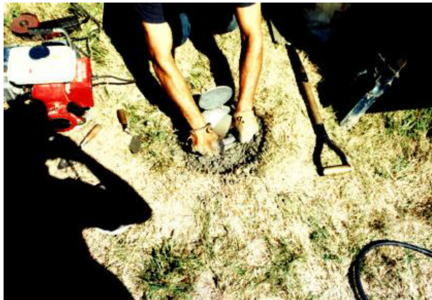
“Shaking” PVC Pipe to Help Settle Concrete
