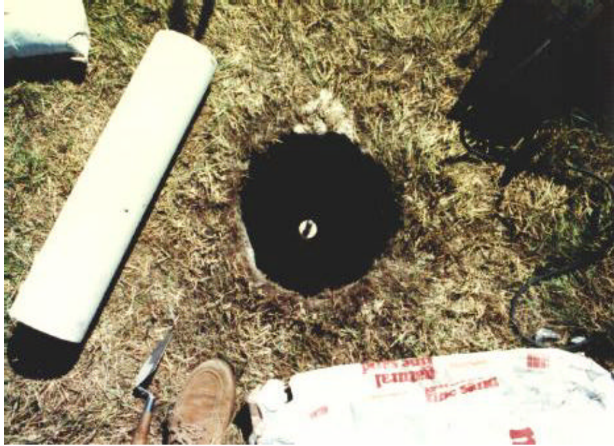
Finished SS Rod and Sand in Place (Note, SS rod centered)
