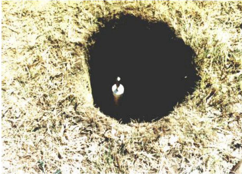
Greased Sleeve in Place Over SS Rod
