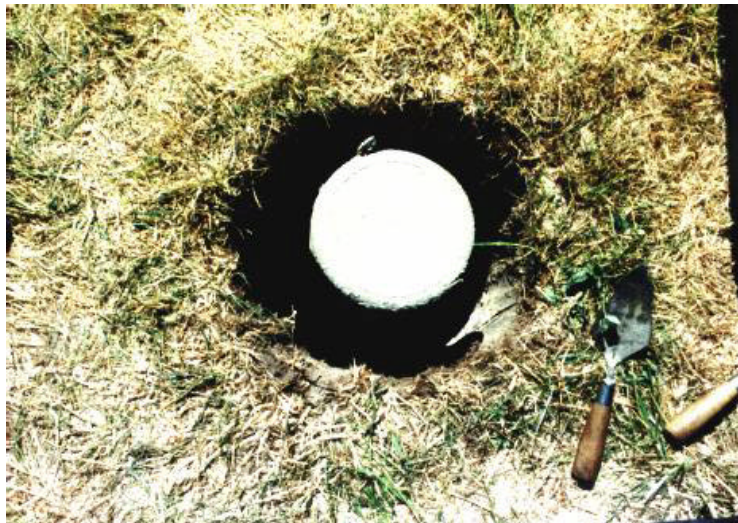
Temporary Cover in Place to Keep Concrete Off Logo Cap
