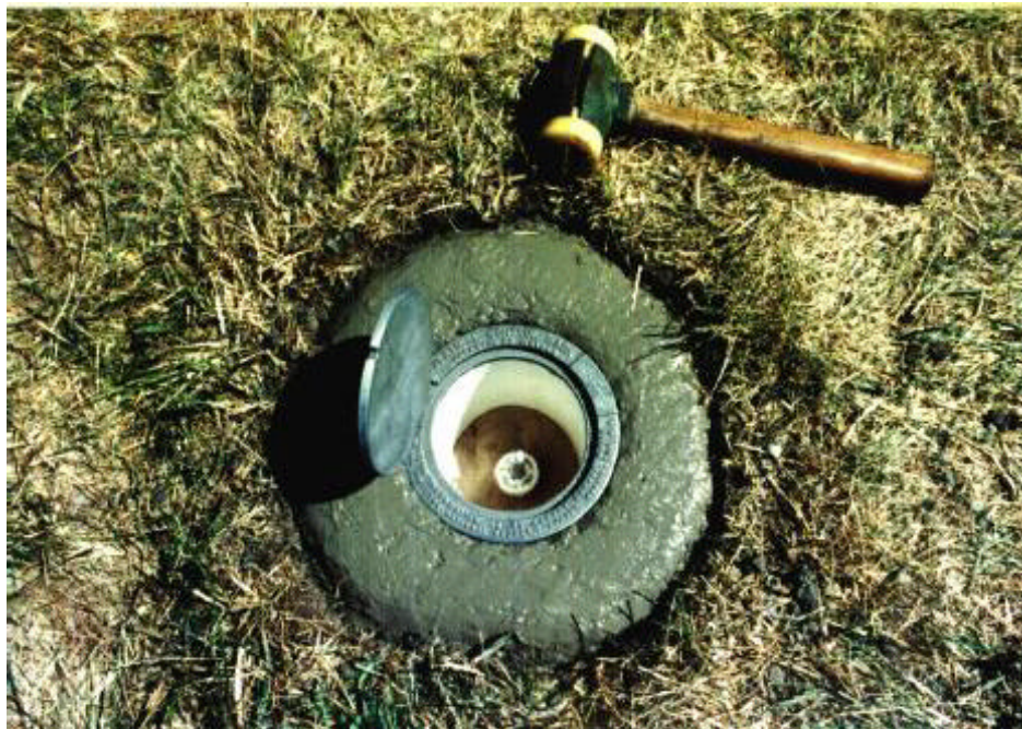
Finished Monumet, Cap Open Note: Very Neat Appearance, SS Rod Centered in PVC, PVC Centered in Concrete, Concrete Round (Not “Mushroom” Shaped), No Concrete on Logo Cap, No Concrete on the Ground
