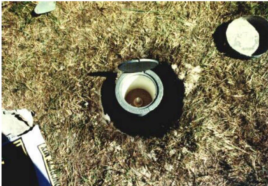
PVC Pipe Backfilled with Sand to Within 1" of Greased Sleeve
