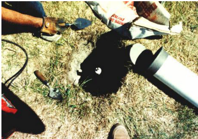
Preparing Hole For 5" or 6" PVC Pipe
