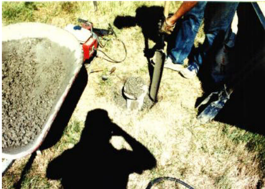
Backfilling Remainder of Hole with Concrete
